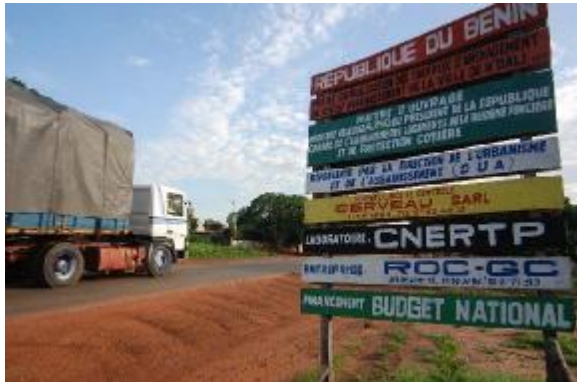
Construction of streets, financed by the "Budget National".
